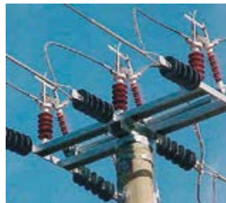
Composite post insulators on an overhead line switch
