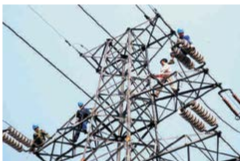
Disc and line post insulators used on overhead lines.
