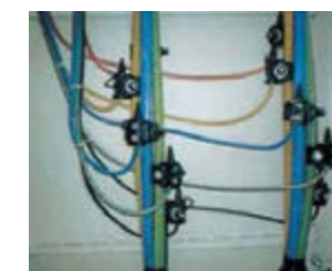
- Piercing effect of wire core
