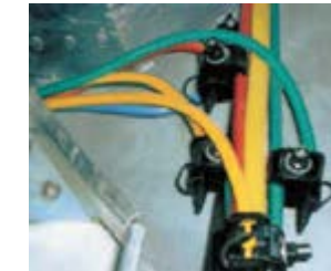
- Piercing effect of insulated coat
